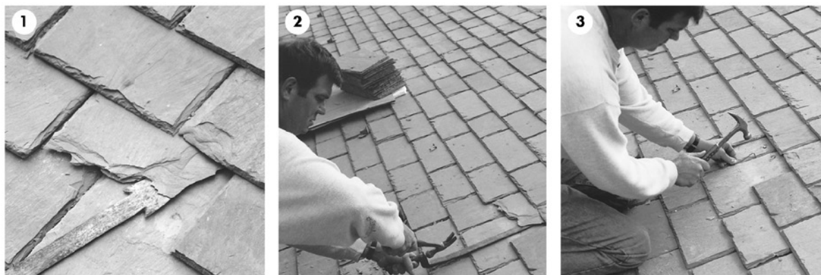
FIGURE B: REPLACING DAMAGED SLATE
