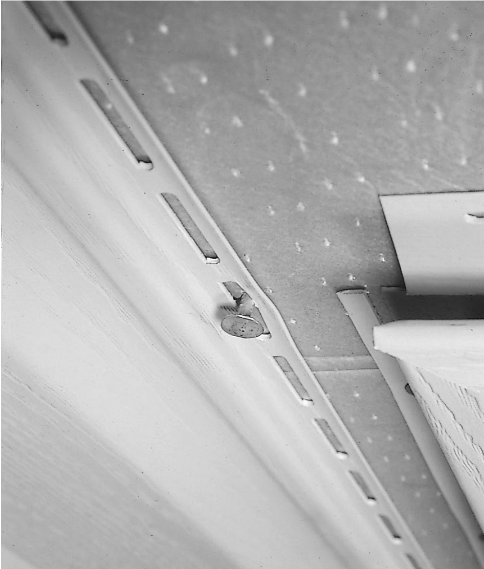
FIGURE: NAILING VINYL SIDING
