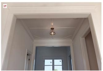
After installing the panels, the author flipped the assembly over and smoothed over the joints with a belt sander (14). A couple of 2x4 deadman supports propped up the ceiling while the crew first nailed and then screwed it through the drywall and into the framing (15). Cove molding covers the joint between the frame-and-panel ceiling and the walls (16). The painted ceiling in the transitional hallway complements the trim in the adjacent entryway and living room (17).
