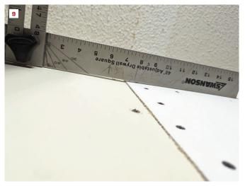
With the backer board positioned between framing members (8), the butt end of a sheet of drywall is pulled in slightly, providing the perfect amount of recess for fast finishing (9).
