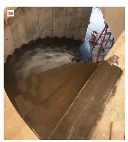
After cutting the rectangular, 2-inch-thick bluestone treads to fit, workers installed them from the top down (14), setting them with landscape adhesive (15). The top tread fit in a notch cast into the landing of the first-floor structural slab so that it would be flush with the porcelain-tile finish floor. All the treads were treated with a stone impregnator and sealer (16).
