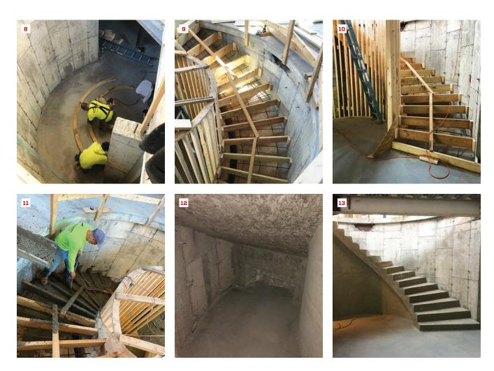
Workers fastened base plates (8) for the two partitions needed to form the stem wall that will support the stairs (9). A third, full-height partition was also built to help form the stair treads, which will cantilever over the stem wall (10). The 4,000-pound, small-stone concrete mix was vibrated carefully during the pour (11). A "safe room" was created under the stairs (12) after the formwork was stripped (13).
