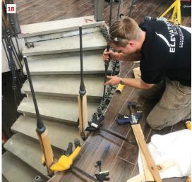
After the baluster brackets were set in place with epoxy and threaded rod, project manager Bryson Gibson used a length of 1/8-inch-diameter wire cable to record the length of the wire-cable handrail and baluster layout (17). Gibson then set up a laser level to establish the tops of the balusters, which were set with epoxy in their brackets and then clamped in place (18) to prep for installation of the wire-cable handrail.
