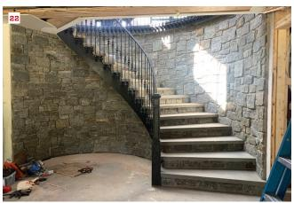
The stripped ends of the wire-cable handrail were inserted into epoxy-filled holes in the newel posts, and held in place with clamps on top of the balusters (19). Then the remaining balusters were installed, with the ends of the balusters welded to the handrail (20). The balustrade was primed and finished with two coats of acrylic coating (21), while natural stone veneer was applied to the risers and walls (22).
