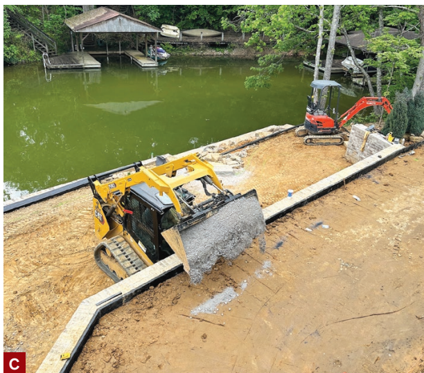
Site work began while the house was still under construction (A). After the infinity edge pool was formed and poured (B), workers began the process of building the retaining walls and backfilling them with gravel and soil to create the two lower terraced levels (C). Here, the crew is installing the stone steps that connect the lowest tier to the dock system (D).
