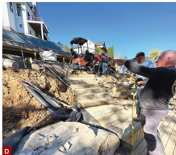
Site work began while the house was still under construction (A). After the infinity edge pool was formed and poured (B), workers began the process of building the retaining walls and backfilling them with gravel and soil to create the two lower terraced levels (C). Here, the crew is installing the stone steps that connect the lowest tier to the dock system (D).
