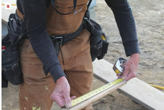
You don't need a pencil to mark cuts that don't have to be perfectly square and a precise length, such as when you're furring out a ceiling or wall with 1x3 strapping for drywall. For longer lengths, just pull a tape and mark the cut with the corner of the tape measure (8). For shorter lengths, use the tape's hook to mark the cut (9).
