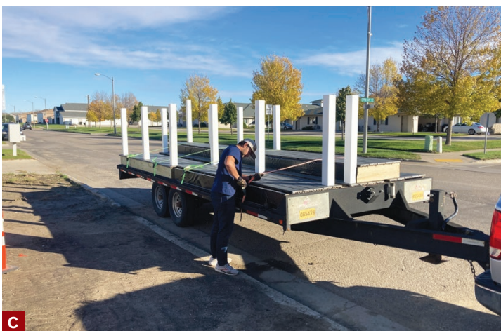
Figure 2. Parts needed to assemble the modules are precut using a TigerStop SawGear automated cutting system (A). Shown here are the modules needed for two decks, with blocking and railing posts installed (B). After the decking is attached to the framing with clips, modules are loaded onto a flatbed trailer for delivery to the site (C).
