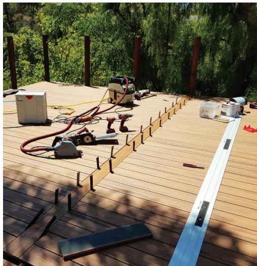
Figure 2. You can avoid the need for butt joints by installing a seam board in the middle of a wide deck. Here, California deck builder Michael Walter used shims to create consistent gaps between the seam board and the ends of the deck boards.
