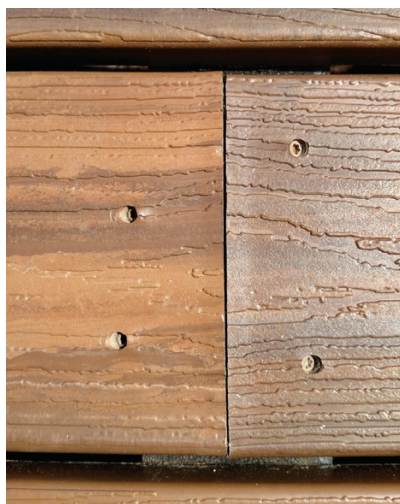
Figure 1. Butt joints in composite decking that aren't properly gapped to allow for expansion can lead to swollen ends (above left). When the break occurs over a single joist, it's impossible to drive fasteners vertically into the joist so that they are perpendicular to the board face while maintaining proper clearance from the ends. Organic material that collects in the gaps between deck boards will trap moisture that can be absorbed by the decking (above right).
