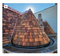
The author special-ordered extra-long, thick shingles that the crew cut at an angle on each side (7). Before being installed, each shingle was hand-dipped into a tub of a borate-based wood preservative. This photo (8) shows the step flashing at the intersection of one turret and the central brick gable. Note the extended copper spout below the limestone capping. A view of the completed roof (9) shows the ribbed ridge caps and soldered copper gutter assembly.
