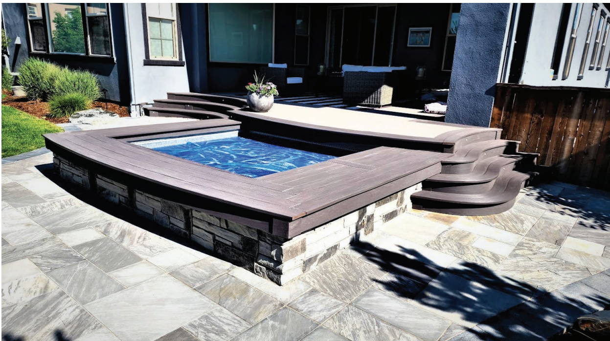
Access to the spa was improved by extending the porch with new TimberTech decking installed over sleepers fastened to the concrete and adding wider curved steps on either side of the spa.
