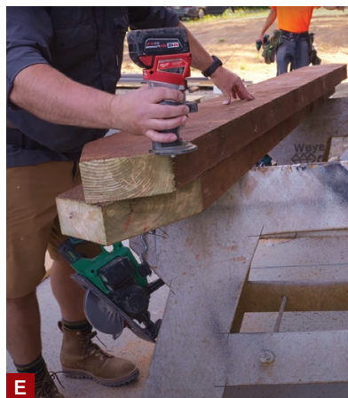
Figure 1. After marking the sawtooth tread-and-riser pattern on a 2x12, the author aligned a mounting bracket and tread block with the bottom edge of the template at each tread location (A), then marked and drilled pilot holes for the mounting screws. At the base, he had to adjust the layout to account for the height of the mounting hardware (B). After checking the fit (C), the author used the template as a pattern to lay out and cut the 4x12 stringers (D), then eased all the edges with a 1/4-inch-diameter roundover bit (E) and applied wood preservative on all surfaces with a roller (F).
