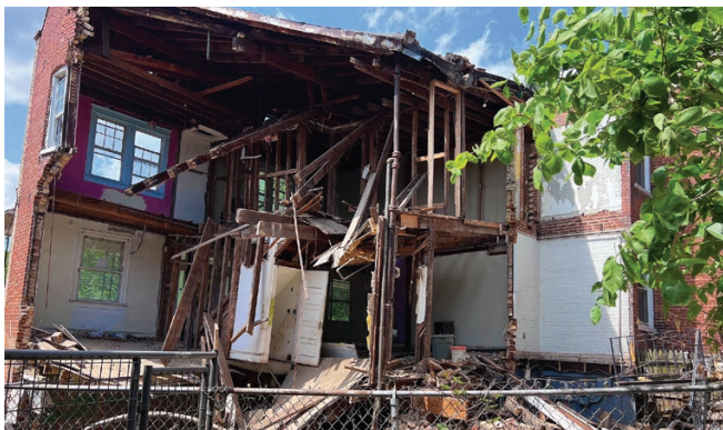
Complete collapse. These photos posted by the D.C. Fire and EMS Department show the tragic consequences of undermining the foundation when digging down a basement.
