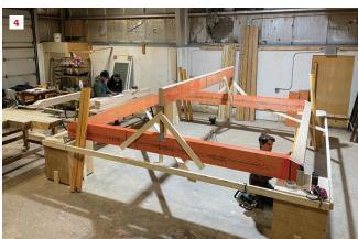
The crew assembled plywood boxes to represent the four columns that would support the roof framing, squared and leveled them, and tied them together with 2x4s (1). Working from a detailed cut sheet (see drawing, opposite), workers prefabricated the components (2), assembled the woven perimeter beams (3), and raised the beveled structural ridge (4).
