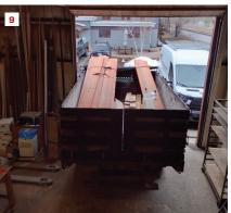
The tops of the LVL hip rafters are beveled (5) and fit neatly into the woven corners of the beveled perimeter beams (6). Raising the assembly a couple of feet above the shop floor made it easy to work on the roof framing (7, 8). After fine-tuning the fit and labeling the parts, the crew disassembled the roof and loaded everything into the back of a truck for transport to the jobsite (9).
