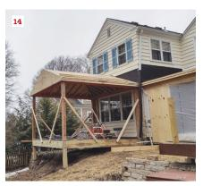
Here, the corner posts have been installed and braced, and the crew has started reassembling the roof, starting with the perimeter beams and posts that support the ridge (10). The gable end wall was assembled on site in two halves (11) to make it easier to hoist into place. Next, the crew framed the eaves on the ground (12), then lifted them into place to complete the roof framing (13, 14).
