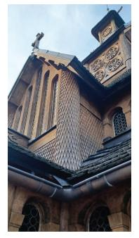
The Kościół Wang, as it is locally known today. is a Norwegian "stave" church dating from around 1200 that was moved in 1842 to Karpacz. Poland. There are no metal fasteners except in the domed copper roof, gutters, and some flashings. Even the wall and roof shingles are doweled in place.
