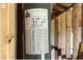
Measure twice, pour once. Solutions for a mis-poured foundation (1) will vary, but the sooner the mistake is identified, the greater the range of options will be to fix it. Check allowable loads. Manufactured pipe columns each have their own rated load-carrying capacity listed on the label. In this example, the center column of numbers shows the allowable loads (2).
