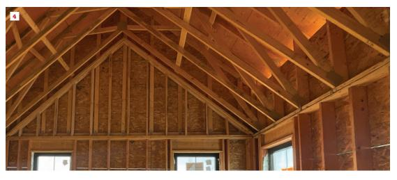
Weak hinge. A stacked gable end wall in a vaulted ceiling creates a "hinge" point in the wall that may provide inadequate resistance to wind loads. To avoid this condition, tall walls should be balloon framed.
