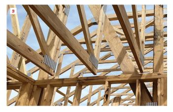
**Check for level at every level.** An out-of-level floor has telegraphed all the way to the top wall plates, resulting in roof trusses that have no bearing.
