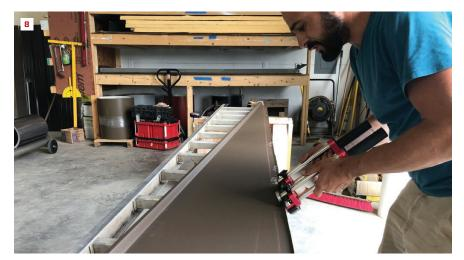
After one of the sections with two female legs had been slit into two pie-shaped pieces, a worker used a roll bender to hand-form first the 1-inch vertical leg (8), and then the <sup>3</sup>/e-inch horizontal leg (9) for the male leg on each tapered panel. In addition to the 34 tapered panels, several full-width standing-seam panels would also be needed to complete the porch roof (10).
