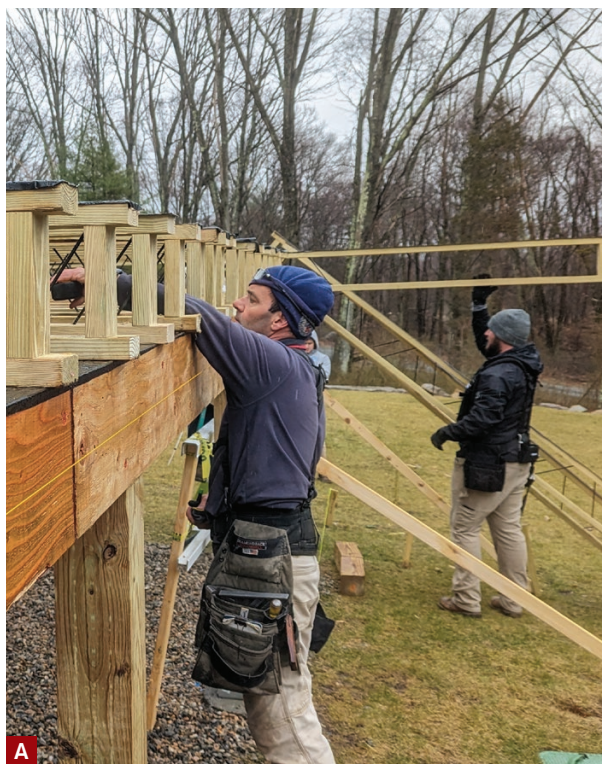
Figure 2. On this project, the Icon joists bear on a two-ply PT LVL dropped perimeter beam supported by PT 6x6 posts, with the top of the beam 1½ inches lower than the bottom of the ledger (A). Once a joist is positioned on the 16-inch-on-center layout, it's fastened to the beam with a pair of structural screws driven down through the bottom chord into the beam (B). Another intermediate dropped three-ply beam provides midspan support and carries point loads from the columns supporting the porch roof (C).
