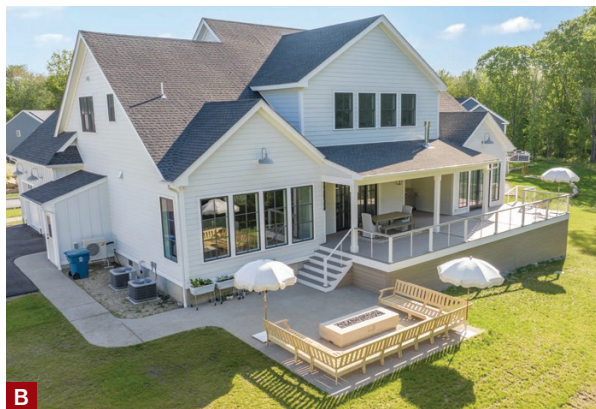
Figure 4. Blocking was also required for the surface-mounted 4x4 rail posts (A). The small landing for the flight of stairs at the end of the deck was conventionally framed and provides access to storage underneath the deck (A). A wider set of stairs at the other end of the deck leads to a poured-concrete patio and sitting area (B).
