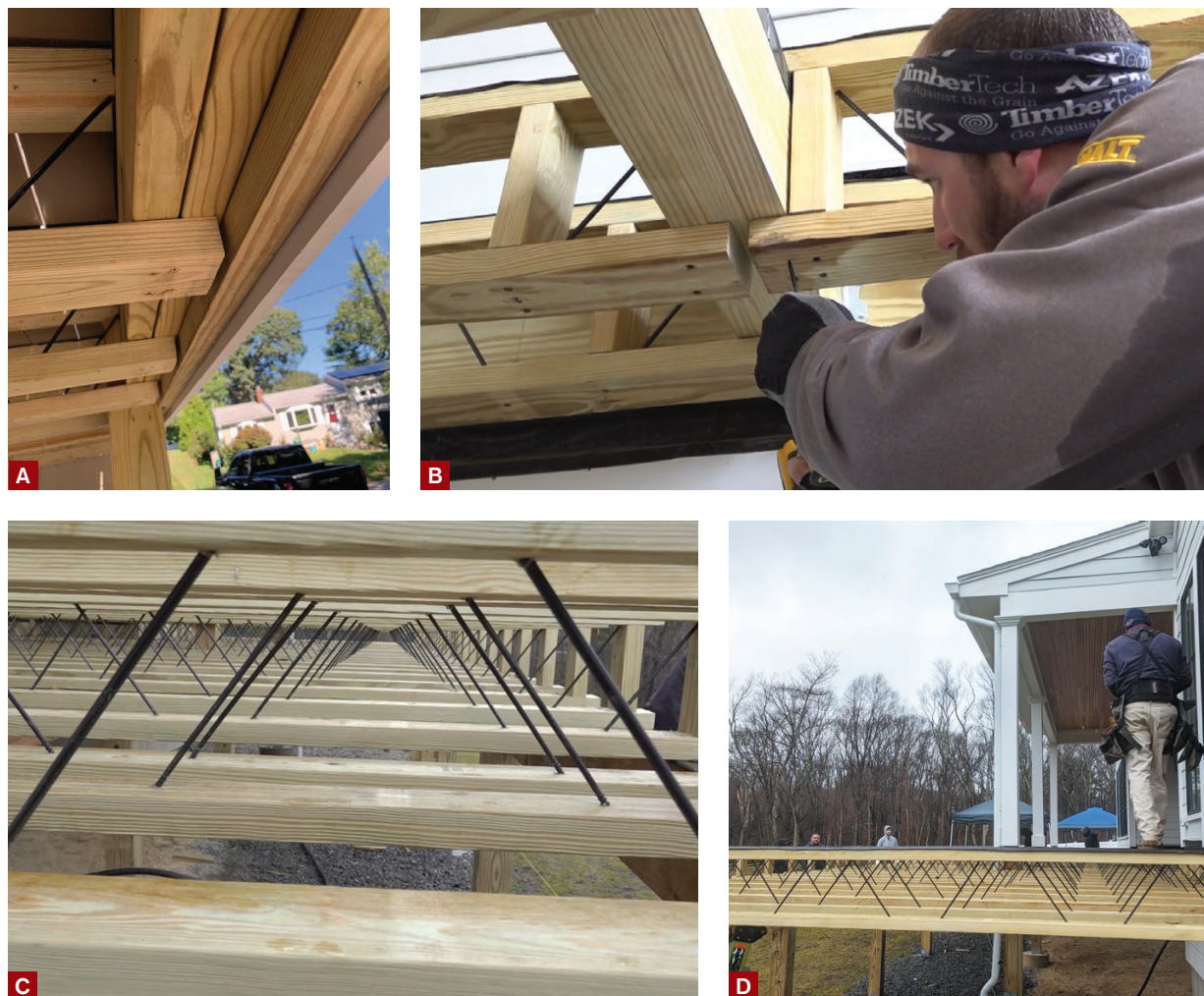
Figure 3. Icon joists can be supported by inset beams as well as by dropped beams. Here, the author removed the squash blocks at the ends of the joists and replaced them with a two-ply 2x8 beam that spans across the support posts, followed by a third ply to strengthen the assembly (A). Inset beams can also be used to preserve clearance under an elevated deck when spans longer than 16 feet are called for (B). Blocking is required midspan and under bearing points but is easy to install because the open web of the joists (C) allows continuous blocking to be inserted from the side of the deck (D). Side rim boards that fit between the top and bottom chords of the edge joists can then be installed.
