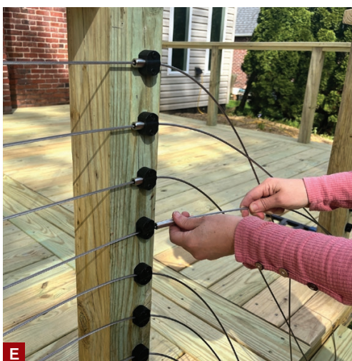
Figure 2. Following the template layout, the brackets are secured to the end posts with two screws per bracket. Next, a “threaded stud spacer” is inserted into each bracket (A). On a worktable, the author assembles a washer and nut on the threaded end of a cable (B). This assembly is fed through the “threaded stud spacer” (C). A flared, unidirectional “pull lock” (D) is then fit onto each cable and pushed into the bracket (E).
