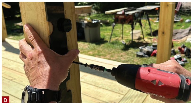
Figure 1. To extend the life of the railing fasteners, the author fastens the top rail to the guard posts from below (A). Between each guard post, he installs a 2x4 subrail (B) to lock the posts firmly in position. This is required to resist the tension the cables transfer to the posts. To streamline the install, he places bar clamps to hold the supplied drilling template to the posts with the bars facing away (C) from where he needs to work with the template (D).
