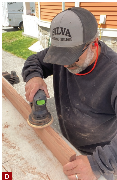
Figure 1. The author ripped a pair of kerfs in the undersides of the 2x4 red balau mahogany rails (A), routed notches in their sides, and then beveled the tops to shed water (C). Prior to finishing, he then sanded them with 100-grit paper (D).
