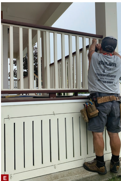
Figure 4. Where upper rails are fastened to the house, the author removed siding and cut back drainage mat, WRB, and board sheathing to install blocking (A). He reinstalled the siding and used a multi-tool to cut pockets for the rails (B), leaving a small gap below for drainage (later, he sealed the tops of the rails to the siding with sealant). The stair railing has similar details, but the nailers aren't beveled, and the rail width is 2 \frac{5}{8} inches for graspability; the ends of the rails and nailers are notched for drainage (D). The author fastened the baluster assemblies to the rails with trim screws driven through oversized pilot holes, which he later capped with Starborn PVC trim plugs (E).
