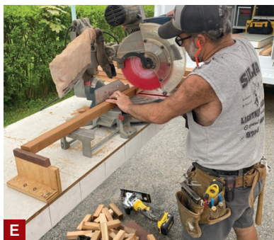
Figure 2. The author applied the penetrating oil finish with a roller, wiped it down after about 20 minutes, then allowed the finish to dry overnight before repeating the process (A). The author made mock-ups of the bottom rail (B) and top rail (C) details to determine the length of the balusters (D). A stop block guarantees uniform baluster lengths (E). Here is the simple jig the author made to safely cut the notches in the ends of the balusters (F).
