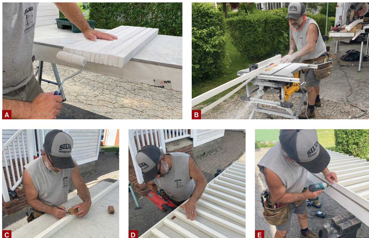
Figure 3. Coating end grain with primer and paint prior to assembly helps prevent the wood balusters from wicking up moisture (A). Here, the author is ripping a 12-degree bevel on one of the PVC nailers (B). After marking the layout from the centers of the upper and lower nailers (C), the author first tacked the balusters to the nailers with 18-gauge nails (D), then strengthened the connection with pairs of 1 1/2-inch trim screws (E).
