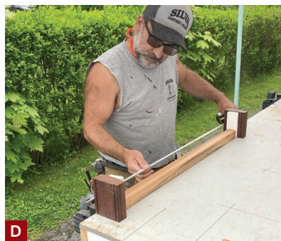
Figure 2. The author applied the penetrating oil finish with a roller, wiped it down after about 20 minutes, then allowed the finish to dry overnight before repeating the process (A). The author made mock-ups of the bottom rail (B) and top rail (C) details to determine the length of the balusters (D). A stop block guarantees uniform baluster lengths (E). Here is the simple jig the author made to safely cut the notches in the ends of the balusters (F).
