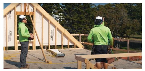
A remote control allows Morton to follow the boom of the telehandler around and physically see what he's lifting from any angle. Having a clean and organized jobsite-the author's Rule #11—helps Morton to move around safely while operating the machine.
