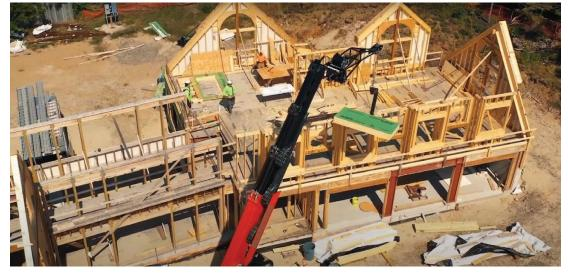
Morton likes to break a project down into the largest liftable pieces possible, then assemble them with the help of a telehandler to avoid working off of ladders. On a large, complex project like this one, having what you need on site when you need it-see Rule #3-is critical in keeping the job moving.
