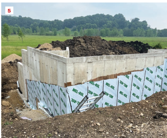
After taping corners and footing-to-wall joints (3), the crew applied sections of membrane vertically to the primed foundation walls (4). The membrane terminates 12 inches below finish grade (5).
