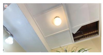
To minimize potential water-leak damage and simplify future projects, the author designs for access whenever possible (1, 2). All the mechanicals that service a remodeled second-story bathroom can be reached from a first-floor half-bath by pushing up on a ceiling tile or by pulling back on the soffit board, which rests on trim attached to the wall and is held in place with removable screws along the outside edge (3).
