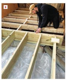
of the scope of work. This meant we had no access to the rim joist and ledger from the exterior. An existing pressure-treated ledger was in good shape, but the rim joist needed to be replaced. To flash the new rim joist, we adhered ice-barrier membrane on new pressure-treated framing material, then flipped it up with the membrane facing the exterior, working from inside the door opening.
