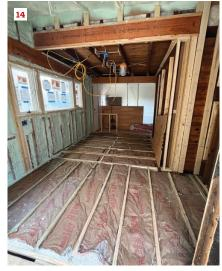
The owner wanted to raise the roof where the old porch roof had been to create a partially cathedralized area (10). There was little existing support at this intersection, requiring a new LVL beam tied into the second-story wall section (11) to support the upper floor and the roof loads (12). This beam landed on top of a new LVL header for new windows (13). Once all the structural work was completed, the exterior walls, roof, and floor were insulated (14).
