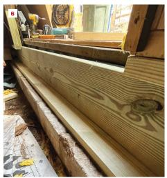
Reframing the floor began with rebuilding the sill where it connected to the deck. After digging out the rotted framing, the crew installed an icebarrier membrane on a new rim joist (5) and then flipped it up to face the exterior (6). While reframing this area, the author set cross-strings to check the plane of the door opening and corrected for a splay in the wall (7). The main house floor was reinforced with sister joists (8), and the old porch floor was completely demolished and reframed (9).
