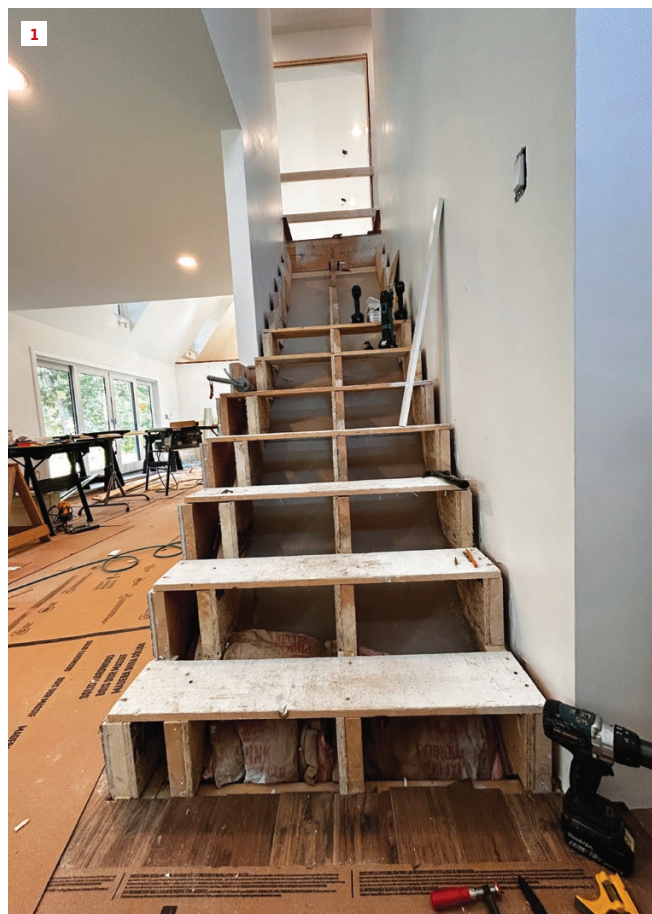
This staircase joining the first and second floors was built with site-made stringers (three main stringers and a fourth, outside stringer) (1). The underside of the stair was drywalled and insulated with batts between the stringers.
