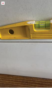
With the baseboard shimmed level, measure how much it needs to drop (1/8 inch here) to match the plinth block. Tack the baseboard in place to set up to scribe (1, 2).
