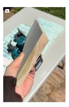
Baseboard can be scribed to fit the floor using a scrap of wood cut to the thickness that the baseboard needs to drop. By running a pencil along the scrap and marking the baseboard, you can see what needs to be removed (3, 4). The author makes the first cut with a planer with a 5-degree back bevel, which makes finer adjustments easier and helps the base sit tighter to the floor, but you can use a table saw or jigsaw instead (5).
