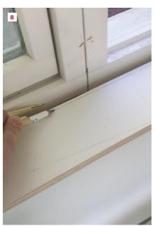
A hand plane works well for final touch-up; alternatively, a sander could be used (6). The trimmed baseboard meets the plinth block as intended with a clean line at the floor (7). Here, a compass is used to scribe a window sill; this technique can be used for baseboard too. Set the compass to the amount that needs to be removed and run the tool as shown (8).
