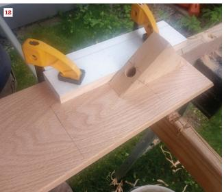
With the story pole clamped in place, lines are plumbed to the wall cap and marked to the handrail (11). By templating, the author could visualize the completed product before drilling finish material. Angle blocks and clamps kept drilling consistent for spindle installation (12).
