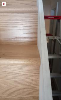
The pants jig (7) the author created allowed him to trace out where the fasteners could be placed for a tight fit of the skirtboard (8). This jig can be saved for future projects. With a lauan template placed on top of the riser, scored lines can be made to match the floor and tread (9, 10). Using a knife to make the lines cuts the veneer, minimizing tear-out.
