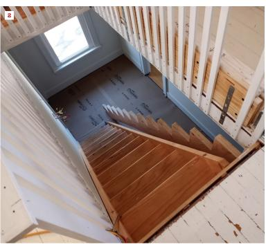
By including all the necessary measurements on a story pole, the author created a layout tool and point of reference for the duration of the project (1). He cut the first stringer and placed it in the opening to confirm fit and make any necessary adjustments. This stringer would be the template for the remaining two (2).
