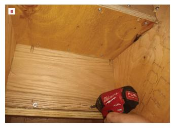
the need for a scotia/cove molding and ensured that the unit run would be exactly the same from tread to tread, even if the stringer cuts were a little bit off. I didn't preassemble the bottom riser and tread, however, because I like to scribe them to fit at the end.
