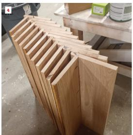
Each tread and riser pair was cut, glued, and pocketscrewed together. Reusable corner blocks kept each assembly square while the glue dried (3, 4). After applying a generous bead of glue, the author fastened each tread and riser pair in place. Predrilling and using truss-head or washerhead screws helps prevent blowouts (5, 6).
