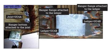
On a deck built after CCA was discontinued for residential use, a joist treated to the level of UC4A did not corrode the joist hanger; however, the ledger, treated to UC4B, caused significant corrosion in less than six months.
