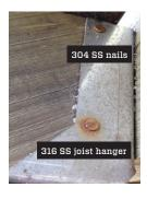
The 304 stainless steel nails are corroding after one year of being near the coast and exposed to chlorides. The 316 stainless steel joist hanger shows no signs of corrosion.
