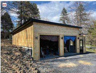
At the top of the end walls, clapboards had to be ripped at a steep angle with a track saw to butt against the frieze board (23). The installed clapboards (24) will be left to weather to gray without any applied finish.
