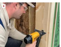
With the garage framed and weathered in (1), the crew prebuilds the jambs and casing (2) for the garage doors using 5/4 #2 pine, easing the edges of the trim using a round-over bit. A carpenter's pencil makes a ready gauge for the casing reveal (3). The bottom ends of the verticals are treated with emulsified wax (4). Using carefully placed 15-gauge stainless-steel nails, a crew member installs the preassembled jamb and casing sets (5, 6).
