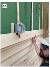
The author uses a simple, site-made jig to align nails precisely so they penetrate only one board (19). Near knots, the crew predrilled for nails (20). A crew member has cut a clapboard to length and holds it in place (21) to mark the precise position for the notch (22) around a wall outlet.
