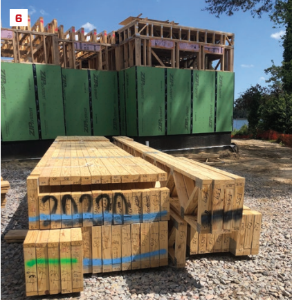
Floor-joist bundles are color-coded after the lumber drop to ensure the correct bundles are lifted to the right locations and oriented in the right direction (6, 7).
