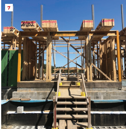
Floor-joist bundles are color-coded after the lumber drop to ensure the correct bundles are lifted to the right locations and oriented in the right direction (6, 7).
