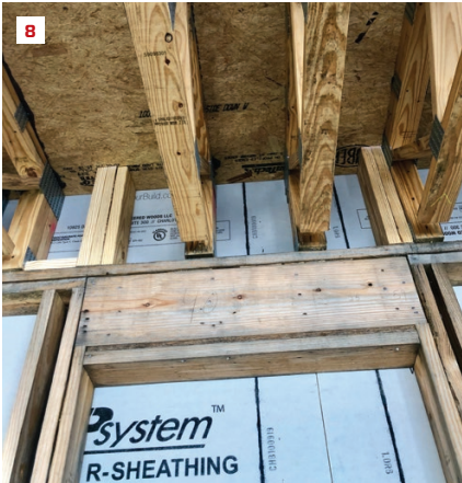
When defining the joist layout, the author's team works off the centerlines of headers and hallways to ensure there's room for can lights (8). Where the gussets of overlapping joists touch, the crew inserts sill-seal foam to prevent squeaks (9).
