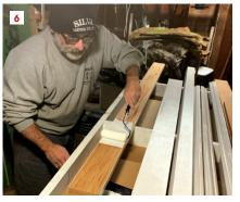
The author removed the old window (1) and replaced it with three new units. He repaired the old framing to be level and plumb or replaced it, if needed. With a new batch of cedar, he modifies, glues, and seals all the trim pieces for the window before installation (2–6). After gluing and screwing the sill together, he bevels it to shed water and cuts a saw kerf in the bottom for a drip edge (5).
