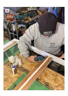
The author cuts the parts to length, pocket-screws them, and glues them together in one step. Note the rabbet cut on the back of the trim to allow for the buildup at the window edge (10).
