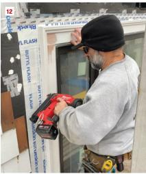
did this a piece at a time to hide some of the screws on the flat stock and to ease transport. The other screws I filled with wood plugs. I then tied in the shingles and prepped for caulking the gap I set between the windows and trim (13).
