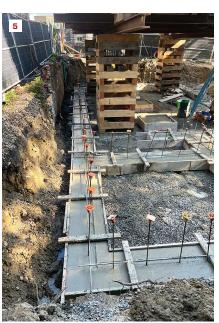
Wherever possible, the house movers located the steel support beams at basement window openings so they wouldn't interfere with the foundation pour (2). The author spray-painted the footing layout as an easy qualitycontrol measure for the formwork contractor (3). Footing forms were lined with GCP Preprufe waterproofing membrane prior to the pour (4, 5).
