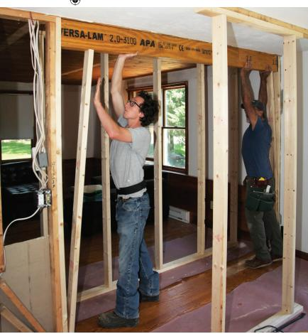
Removing part of an interior bearing wall to create an opening less than 12 feet long with a direct load path to the foundation is a straightforward condition that most competent builders can handle on their own. However, on the job shown here, an engineer provided by the LVL supplier verified the beam size and bearing requirements—welcome guidance for the builder.
